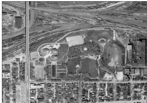
Construction Complete on the Domes, 1967
