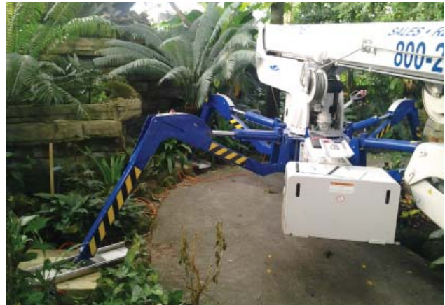
Specialty lift used to maintain the Domes
