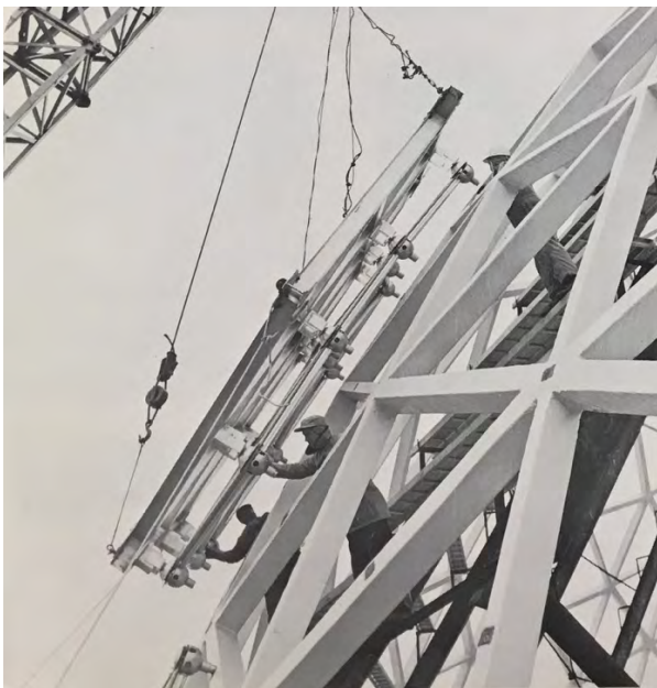
Figure 4 Photograph showing a pre-assembled glass panel being lifted into place. The hubs connect the glass to the concrete at designated points (dark squares). (Printed in Mitchell Park Horticultural Center guidebook ca. 1968)
